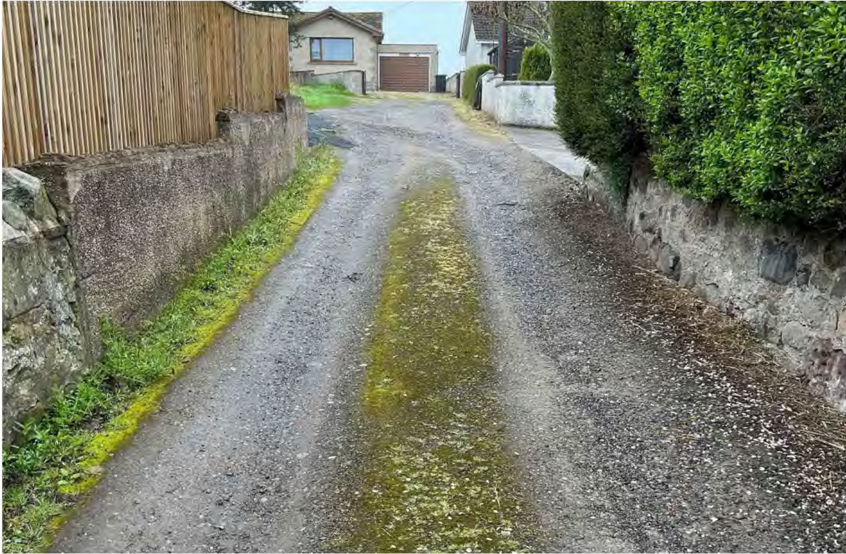
Figure 4. Access Road as of May 2023
